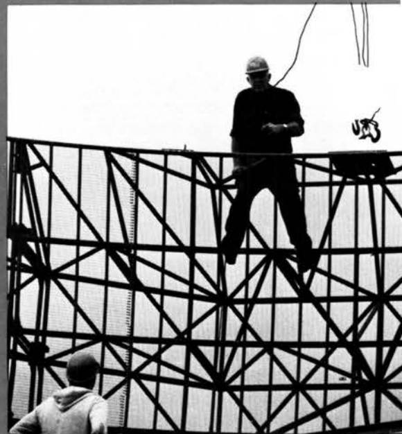
STRIKING A BEACON —NAFEC equipment operator Robert Brooks attaches a hook to a radar beacon antenna for dismantling. The experimental antenna was tested, then returned to the manufacturer, prior to further NAFEC testing.
