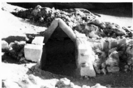
The beginning of a snow shelter with an un-keystoned arched roof and, at right, the finished snug survival domicile.
