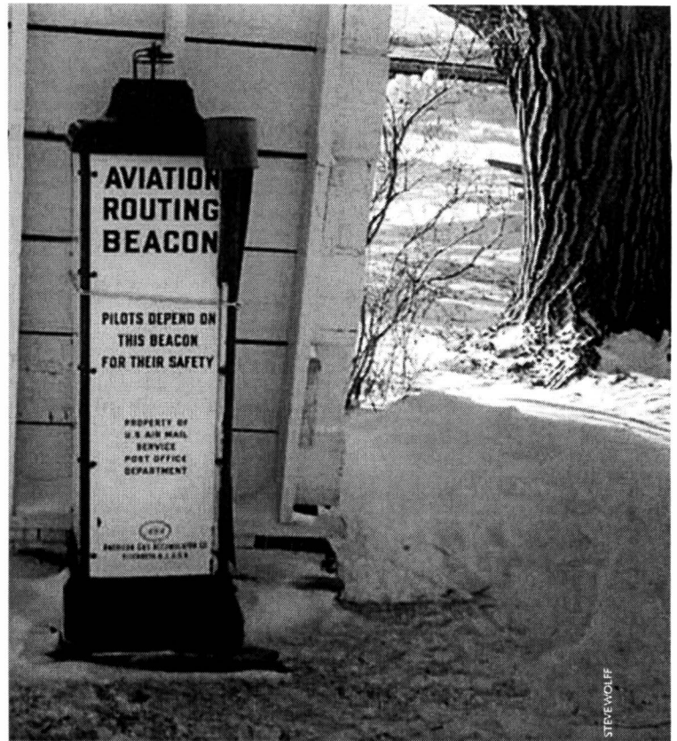
AGA cabinet beacon powered by acetylene gas without a 6ft pylon on top. Classed as ARB (acetylene range beacon), these small beacons had a 300mm dioptric lens at the top of the pylon and blinked 60 times per minute. They were installed every 3m where terrain obstructed the view of larger towers
