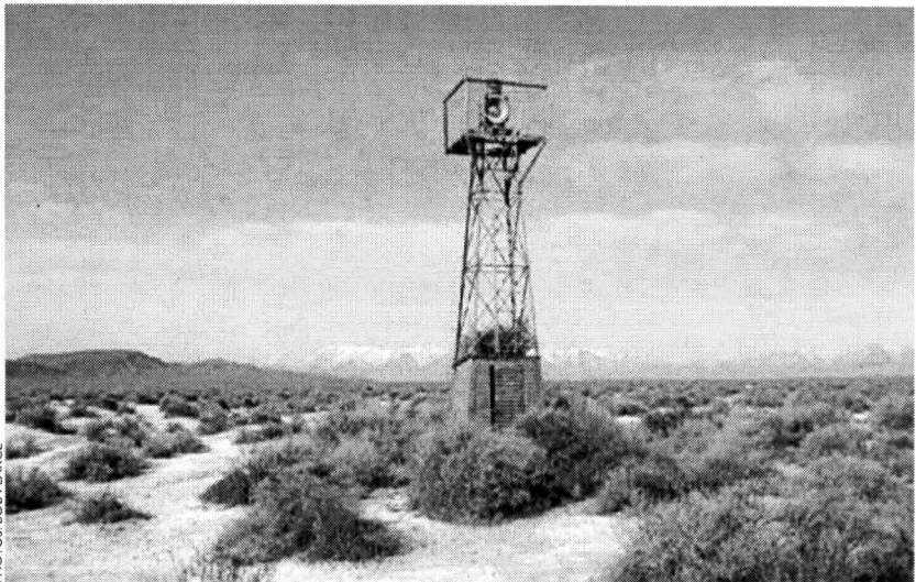
Site 29 on the SL-O airway in the mid-Twenties. A 24in beacon with two course lights—green in this case to denote the presence of a landing field. The small building with '29' painted on its roof is the power house. Large house with 'DANA' on the roof is for the airway keeper.
