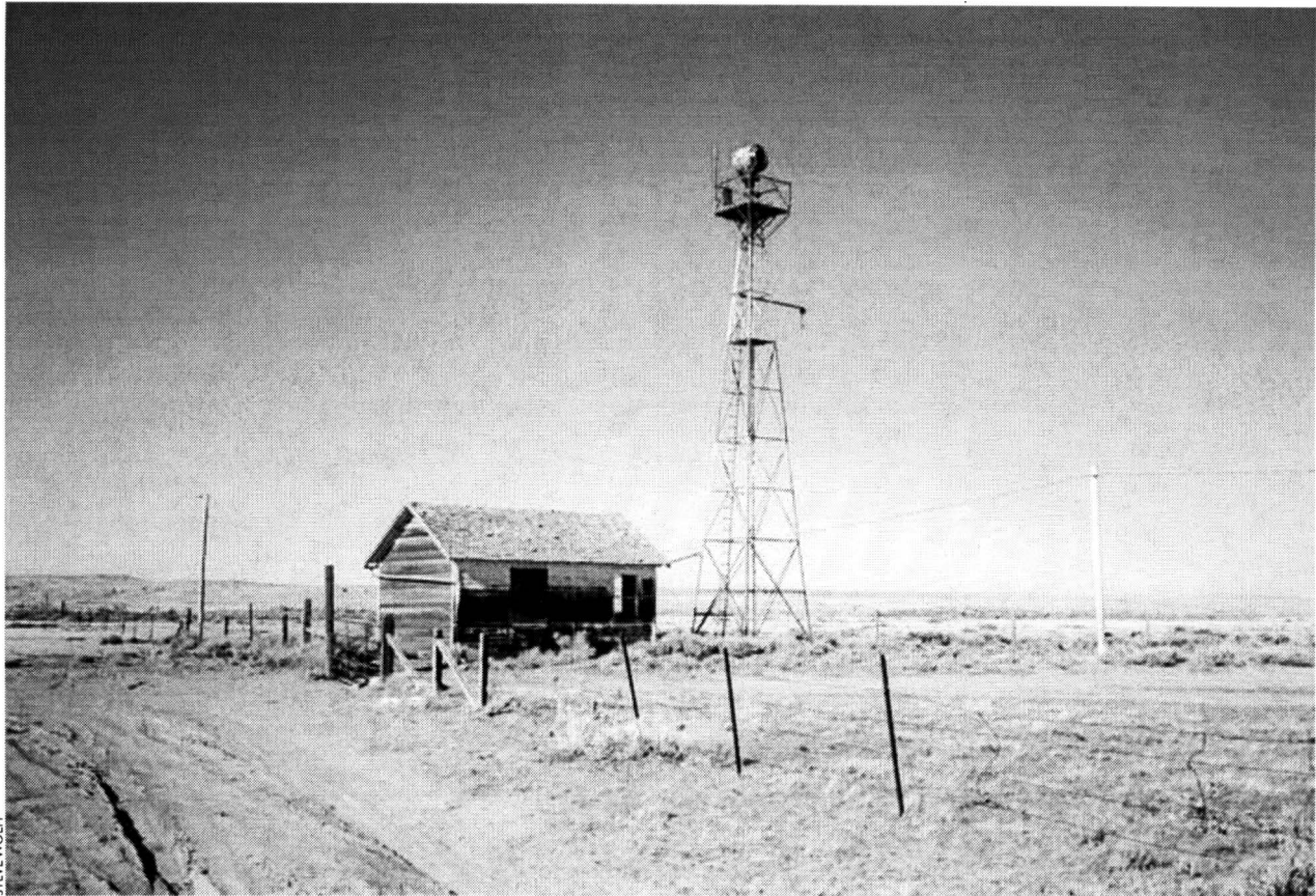
Surviving Thirties-era beacon at Site 32 on the SL-O airway, upgraded to a 36in double-ended style, without course lights and fuel tanks. Beacon was now classified as Type D standard beacon at intermediate field using AC commercial power.
