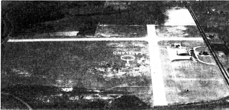
FIGURE 21.—Air marker constructed of white lime rock and imbedded in the landing area.
