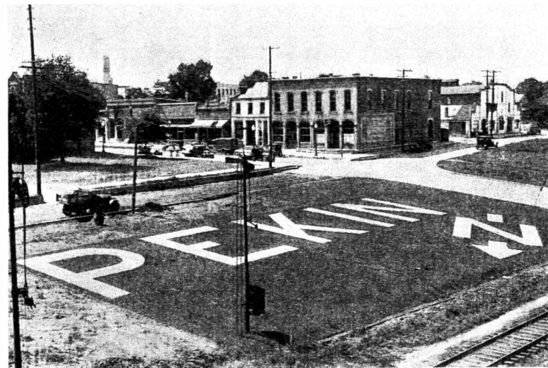
FIGURE 19.—Air marker constructed of concrete adjoining a railroad station. Marker shows name of community and meridian pointer. Abbreviated name of the State should be included. Note excellent maintenance of marker and sod background.
