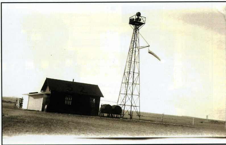
Photo 5: The wind sock on the tower, or “Dad’s pant-leg”. This also shows the office before it was painted., c.a. 1930.
