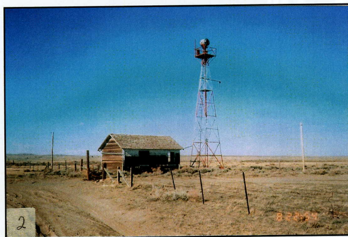
Photo 32: Looking NE at office and tower. Below the tower is the arrow pointing to the next station. To the right (east) of the tower, about 1,500 feet, was the range consisting of five poles with an antenna strung between them in the shape of an X.
