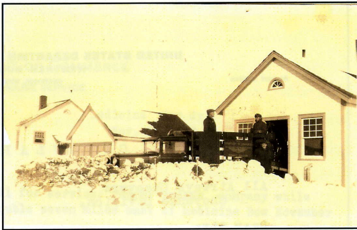
Photo 18: This shot of the power house was taken before the elevation numbers were painted on .
