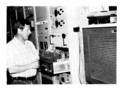
At the Baton Rouge Sector Field Office, electronics technician Richard Stanton performs a check of the instrument landing system remote monitor.
