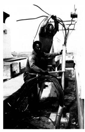
Resident engineer Les Thomas (foreground) and marine machinery mechanic Phil Bourgeois run cables to the standby engine generator at the New Orleans Lakefront tower under construction.
