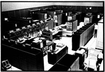
Automation in NAS Stage A meant a computer complex like this prototype at the Jacksonville ARTCC in 1967.
