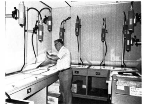
For the Model 1, Bridgeport specialist Richard Kniat positions facsimile weather maps under closed-circuit TV cameras that feed TV monitors at the pre-flight, in-flight and NOTAM Positions.
