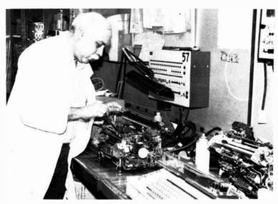
Peripheral device technician Harold Taubes adjusts a flight strip printer in the sector's repair shop.
