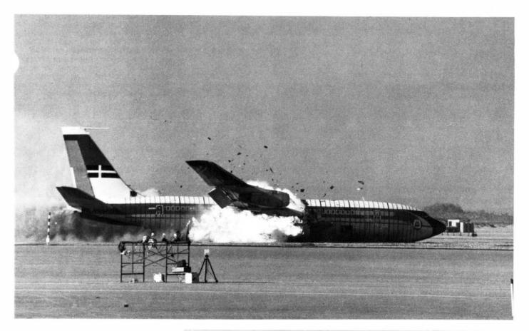
A fireball erupts as one of the cutters severs the fuel line between degrader and engine, spilling burnable kerosene instead of the stored treated fuel.
