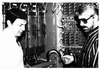
John Cotter, environmental systems engineer, and Bob Williams, environmental support technician, align the new power conditioning system for the Memphis airport's radar.
