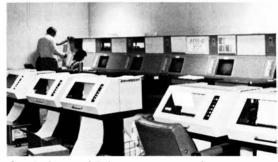
Jim DeBerry of E-Systems, Inc., and Sandra Mahlberg from the Chicago ARTCC help perform system shakedown of the Flight Service Data Processors (FSDP) at the Automated Flight Service Station position consoles and line printers at the FAA Technical Center. The FSDPs are now being installed at the Cleveland, Ohio, ARTCC to serve the Cleveland; Dayton, Ohio; and Bridgeport, Conn., AFSSs.
