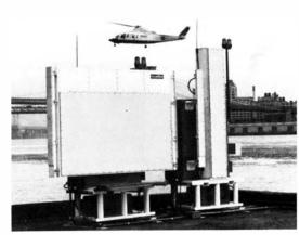
An FAA helicopter makes a demonstration flight to the microwave landing system-equipped Wall St. Heliport in New York City. Only a heliport has the elevation and azimuth antennas collocated. The agency presently has 170-plus MLSs on order, including systems for three heliports.
