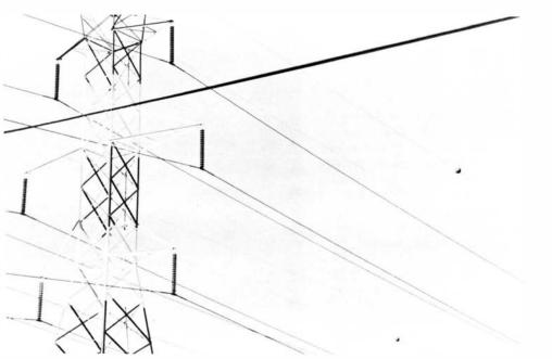
Orange globe markers are used to call pilots' attention to otherwise invisible high utility powerlines in the path of takeoffs and landings.
