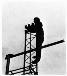
Replacing an obstruction light on the glide slope antenna at Scottsbluff County Airport is electronics technician Joel Myhre.
