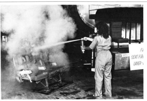
A Tech Center employee extinguishes an airline seat fire with a new Halon 1211 extinguisher which does the job faster and at greater range than other types.
