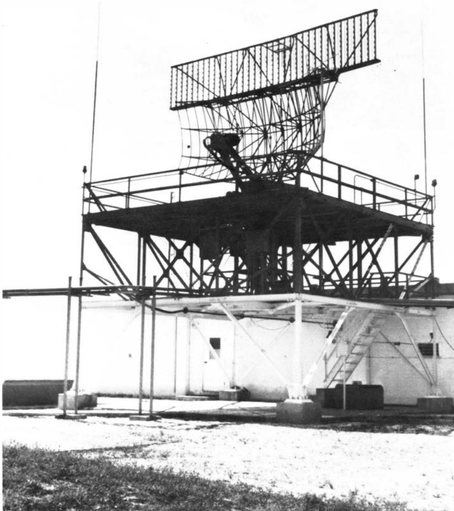
This is the antenna for the Third Generation: The five-foot open array atop an ASR-7 provides improved beacon performance and makes possible the Mode S capability for data link.
