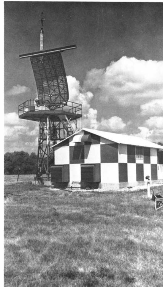
Airport surveillance radar came in earlier than long-range radar. This ASR-3 was already being supplanted by the ASR-4 when photographed in 1961.
