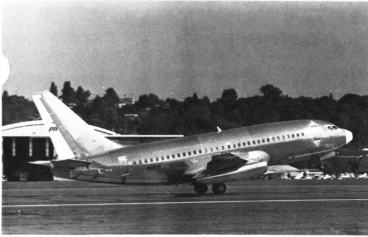
In 1980, Boeing tested this 737 with a graphite-epoxy composite horizontal stabilizer, which weighed 22 percent less than the conventional structure. Boeing photo
