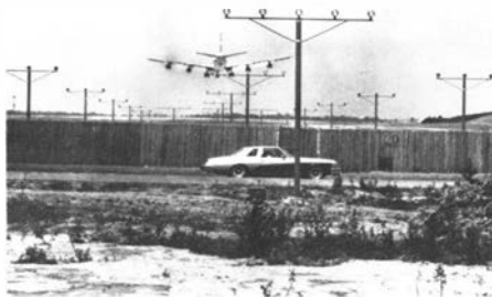
To make approach lighting less dangerous in a crash landing, rigid support structures were replaced with frangible ones.
