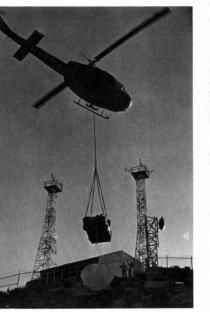
Another load of materials is delivered to the mountaintop, with a drogue parachute to stabilize the load.
