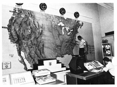
the 48 states that can provide more information about the missing aircraft. A primary tool here is the Interim Track Analysis Program (ITAP). With a last known position and time for the missing aircraft, an ARTCC data systems specialist at 15 of the 20 centers can run a computer program that will generate a printout of an aircraft track based on its radar return. This is a projection based on information retrieved from computer tape recordings of all radar data of the time in question.
