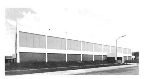
A windowless exterior and an earthen berm covering the lower portion of the walls are among the elements of the new energy-efficient Radar Training Facility that has risen at the Mike Monroney Aeronautical Center.
