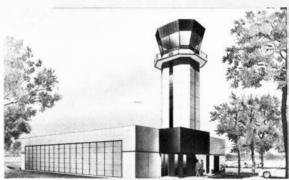
The Golemon & Rolfe design for today's intermediate-activity facility combines a non-functional shaft, surmounted by an eight-sided cab, with various sized base buildings erected according to need.
