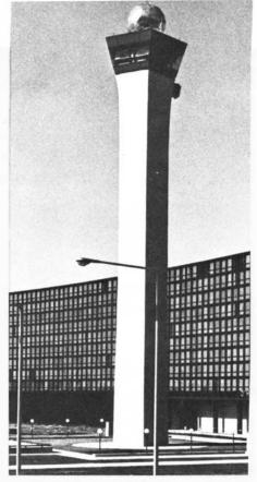
I.M. Pei designed 22 of these pentagonal towers—O'Hare's shown here. Non-cab functions are below ground. The shaft's graceful lines are broken by only a permanent track-mounted window-washing bucket, which was recently replaced by a catwalk, permitting the job to be done better.
