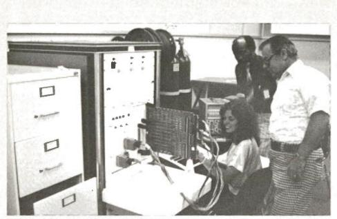
**RADAR BACK-UP IN PLACE**—Electronics technician Bob Hayes (right) shows technician trainee Sue Leech the operation of the Direct Access Radar Channel (DARC) printed-circuit-board tester recently installed at the Minneapolis ARTCC, while John Smith of Raytheon observes. A replacement for broadband radar, DARC will be undergoing shakedown tests at the Salt Lake City, Minneapolis and Chicago en route centers.
