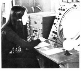
With her left hand in the equipment drawer, radar technician Peggy Post adjusts a maintenance scope serving the Wichita Tower.
