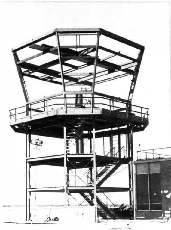
**SORT OF SHORT!**—This abbreviated tower going up next to the Atlantic City terminal is really a NAFEC test bed for tower mockups, previously created inside center buildings. Art Holmes monitored its construction.
