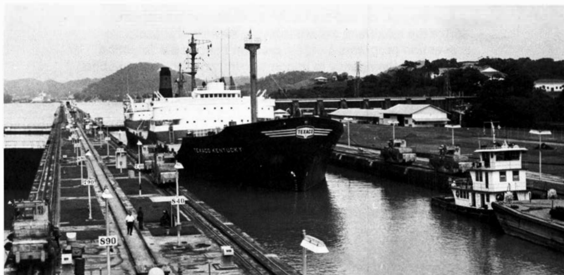
A tanker moves through the miles long Miraflores Locks en route from the Atlantic to the Pacific. These locks raise or lower ships in two steps a total of 54 feet.
