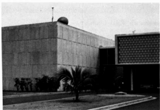
The FAA headquarters at Balboa houses the area manager's office, the CERAP and the IFSS. It was built in 1962.
