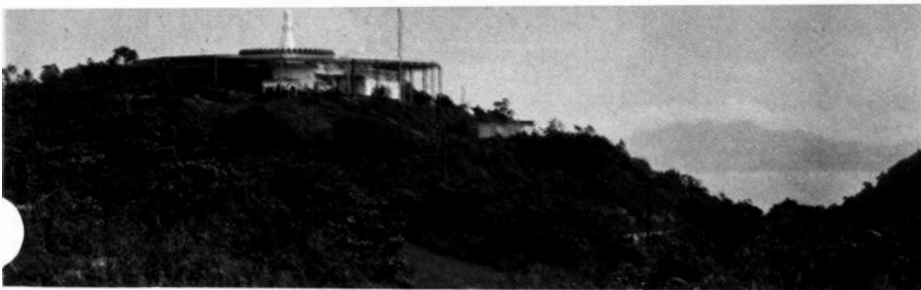
The VORTAC sits on the highest point of Taboga Island, 999 feet above sea level. FAA technicians commute by boat every day from Balboa—a 14-mile trip.
